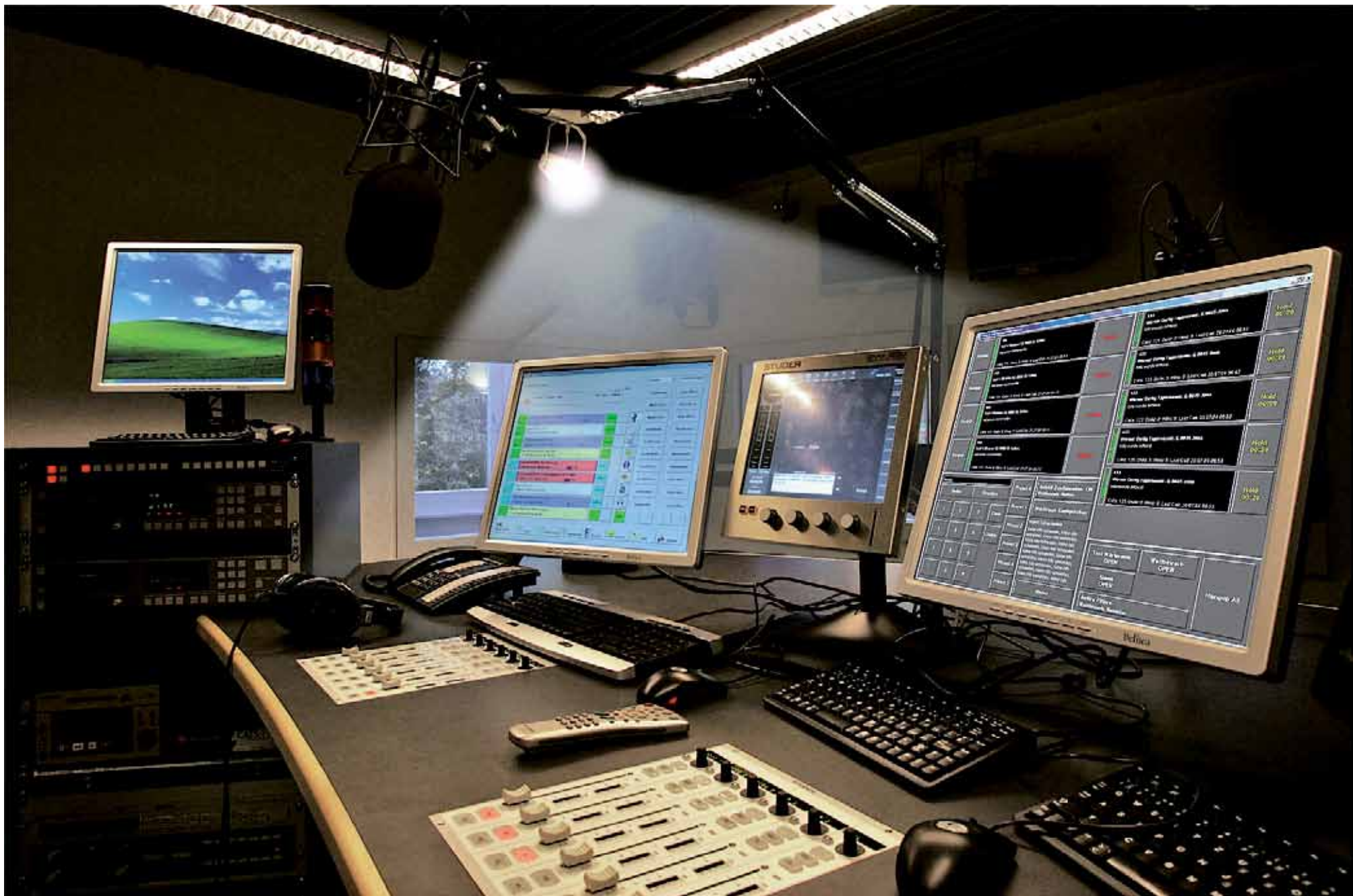
Switzerland, Radio Zürichsee, Rapperswil, OnAir 3000 Modulo
