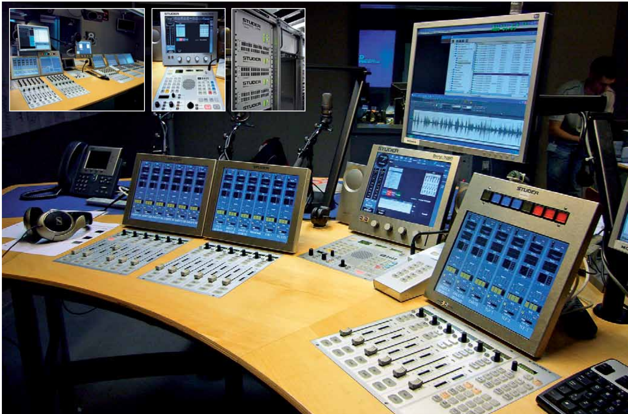
Denmark, Danish Radio Copenhagen, OnAir 3000 Modulo
